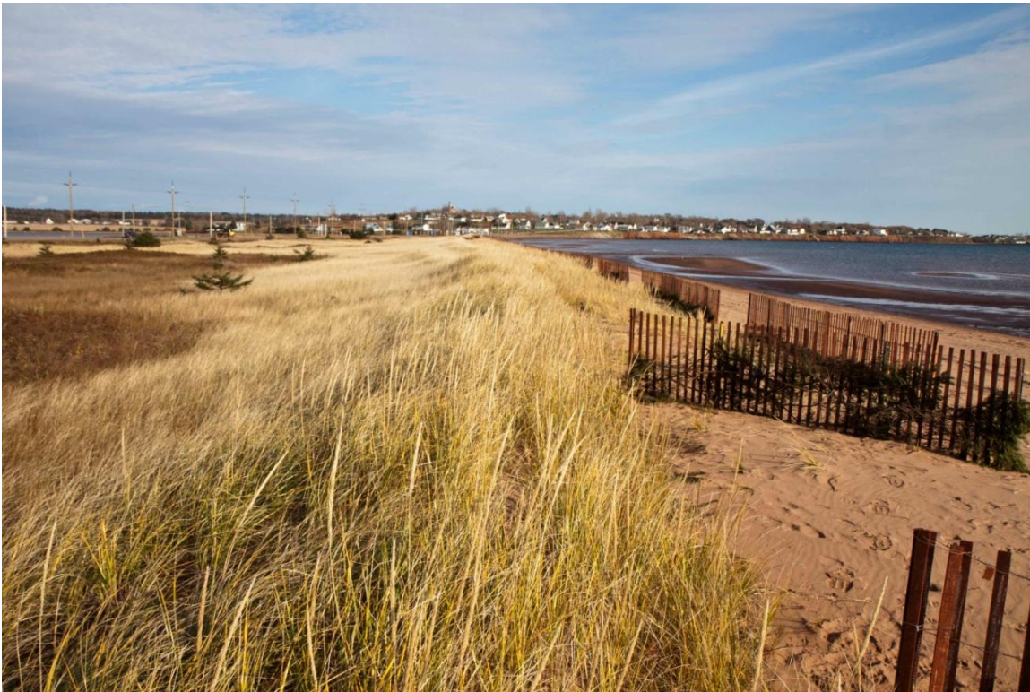
PHOTO 17 - DUNE PROTECTION CONSISTING OF SAND FENCE WITH SPRUCE BOUGHS, SOURIS CAUSEWAY, P.E.I. (PHOTO CREDIT D. JARDINE)
