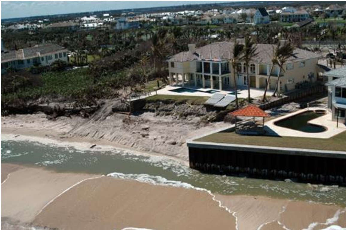
PHOTO 15 - SEA WALL IN DOTHAN, ALABAMA ACCELERATES EROSION ON ADJACENT PROPERTIES (PHOTO CREDIT ADVANCED COASTAL TECHNOLOGIES)
