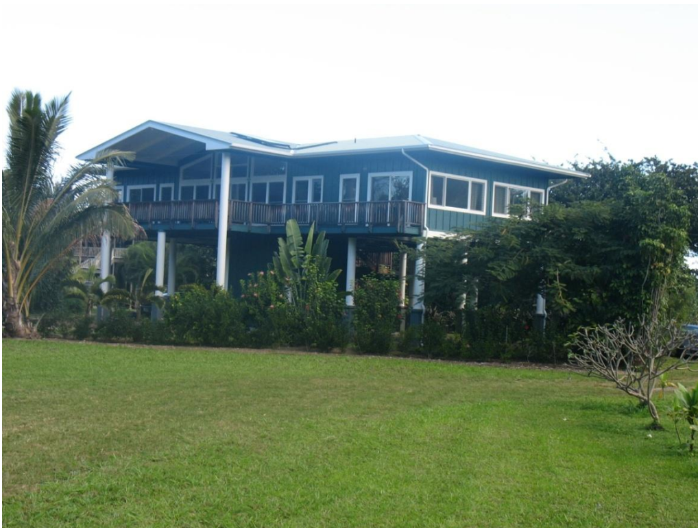
PHOTO 11 - WATERFRONT HOUSE 3 METRES ABOVE GROUND ELEVATION ON NORTH SHORE OF KAUAI ISLAND, HI (PHOTO CREDIT GRAHAM FARSTAD)
